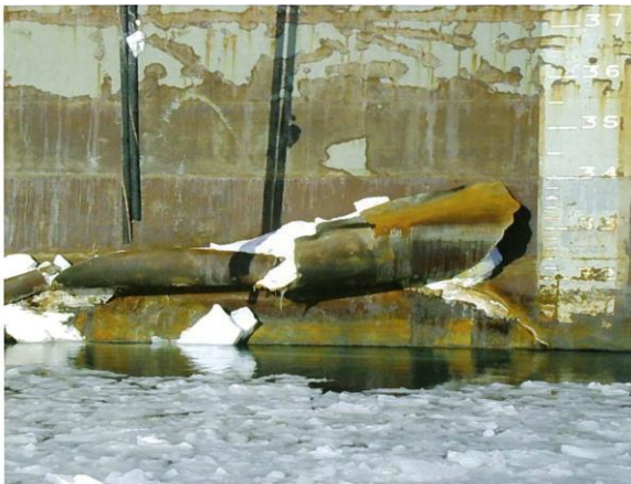
Figure 1. Collapse of ice protection belt at "Molikpaq" platform (Vershinin at al. 2006)
