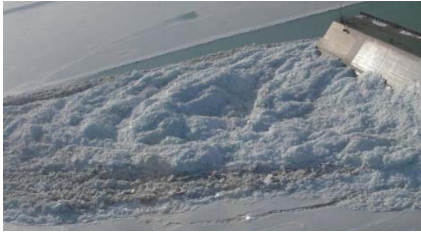
Figure 1. Rubble build-up against a steel ice protection structure in North Caspian Sea
