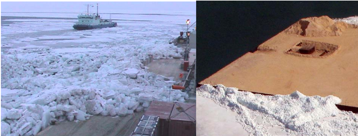
Figure 1 Examples of ice encroachment at structures in the North Caspian Sea
