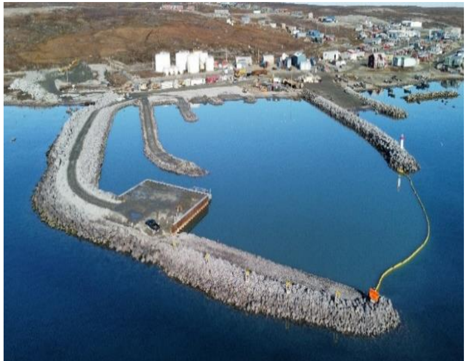
Figure 2. Clyde River SCH, under construction September 2024. Dredge haul roads still in place.
