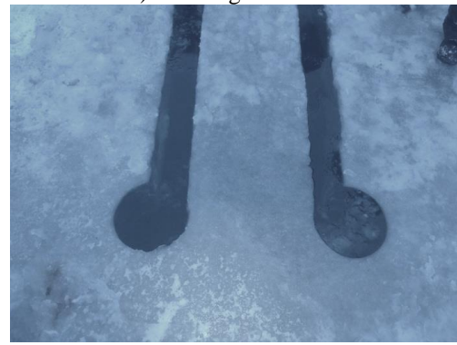
d). Beam root with 200 mm holes
