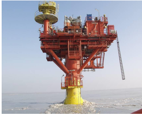
Figure 2. The JZ20-2 NW conical jacket platform
