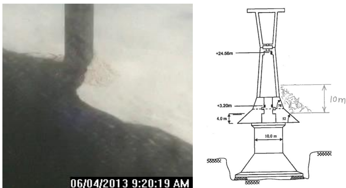
Figure 4. Ice conditions at pier 23 during the maximum loading event on April 6 th , 2013
