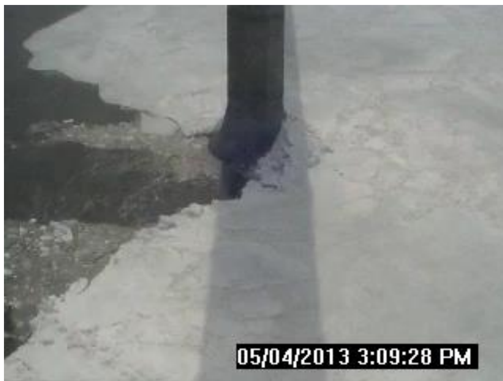
Figure 6. Ice conditions at pier 23 during the maximum loading event on April 5 th , 2013
