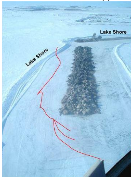
Photo 2. Completed rock pile with crack markings in foreground; rock pile construction in background
