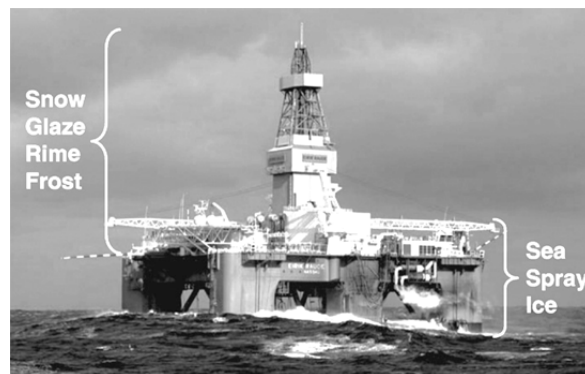
Figure 9. Potential ice accretion areas by ice type on a platform (Paulin, 2008)
