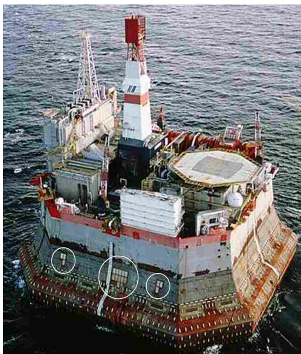
Figure 1: (Top) Ice load panels installed on the north face of the Molikpaq structure. (Bottom) Molikpaq during tow at a low draft. The three groups of pressure panels (N3, N2 and N1) are encircled.
