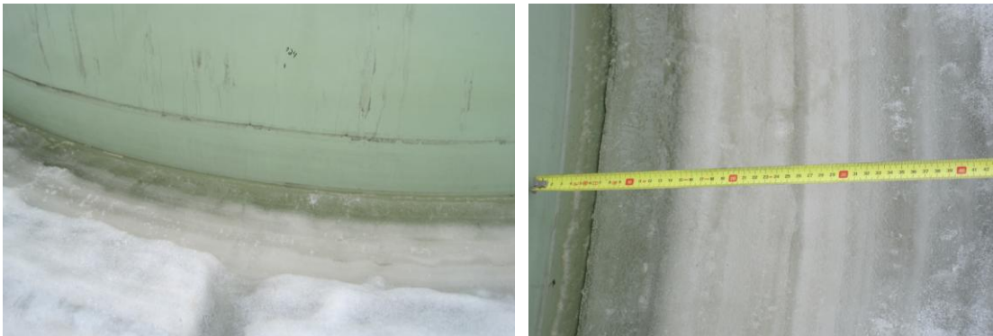
Fig. 6a) and b) The effects of slow ice movements and temperature changes. (6b scale: red spots 100 mm)
