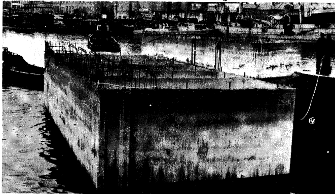
The caisson is towed.
