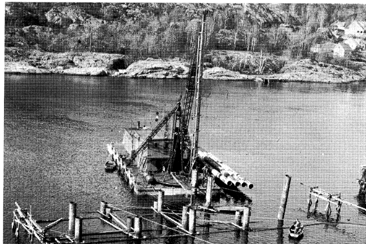
Steel pipe-piles - reinforced and concreted as pillar (Framnes, Sandefjord) and the 7 m/m steel pipe can be regarded as "ice-skin"
