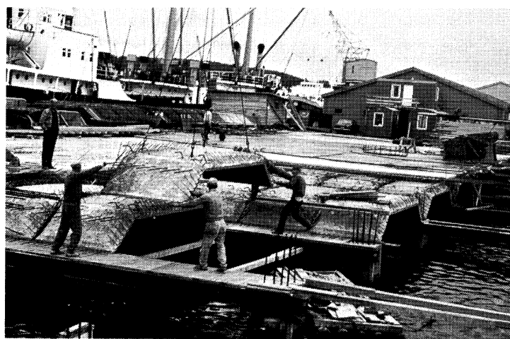
Pre-fab quay slabs - Placed
